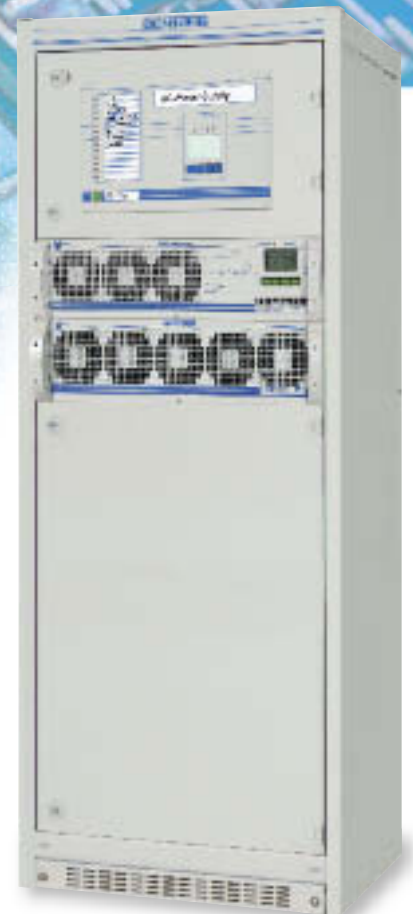
Fig. 7: Inverter cabinet with 8 inverter modules, static and manual bypass. Total AC output power 12 kVA
